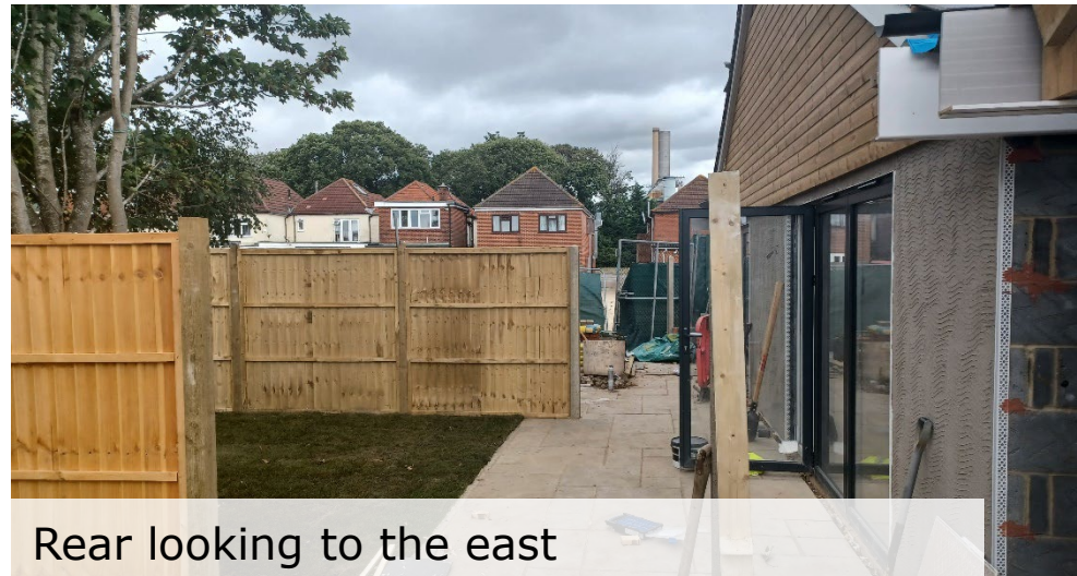
Eastern end of site
